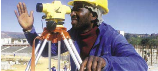
A surveyor works at the construction of the Bafokeng Stadium in Rustenburg. The acquisition of intermediate artisan and technical skills for infrastructure development is a short-term objective of JIPSA. Photo: David Gossard/South Press/The Big Picture
